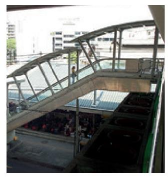
Figure 4.3 The outdoor escalator should be covered by a roof to improve passenger safety and convenience
