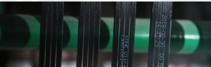
At 110 North Wacker Drive, that means dramatic energy savings. Based on 300,000\* starts annually, we estimate that energy consumption in each of the eight high-rise elevators and two high rise service elevators using KONE UltraRope® was reduced by 35 percent compared to elevators using conventional steel rope.
